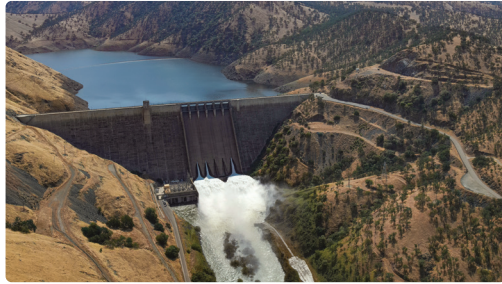
Pine Flat Dam low level gates releasing water into the lower Kings River, May 2023.
