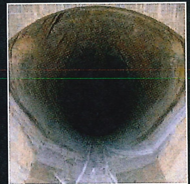
Pipes and Culverts
