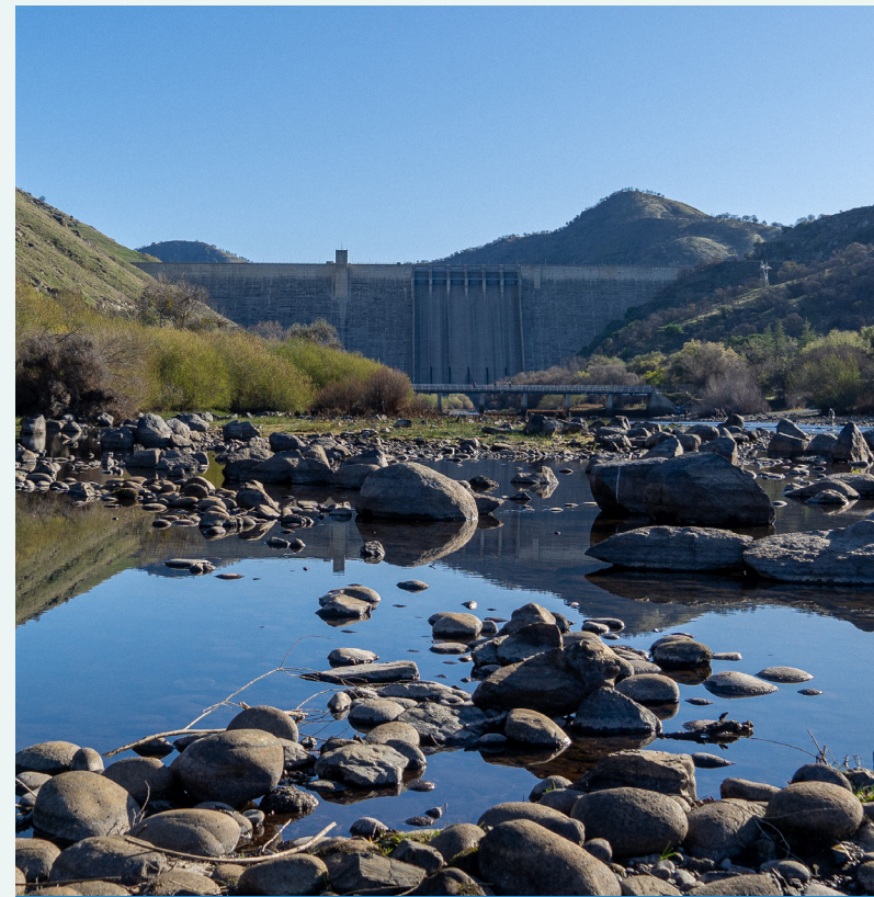
The Kings River beneath Pine Flat Dam shows low water levels, exposing parts of the riverbed normally under water.
