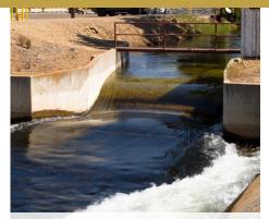
The most common type of open channel canal measurement used by FID is the Replogle Flume, such as the one shown here installed on the Gould Canal.
